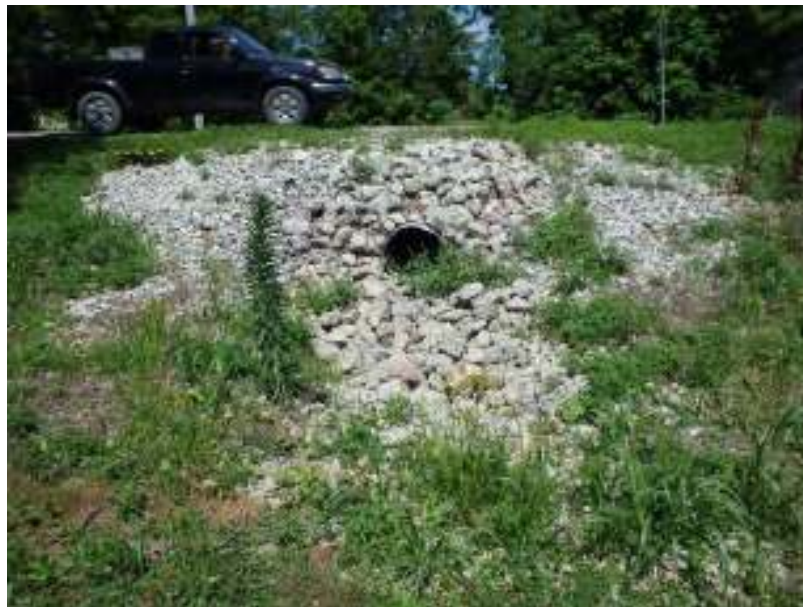
PP6 – Looking at pipe and riprap on E side of Blaine Pike
